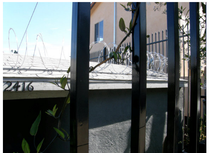
Razor wire on roof at rear.
