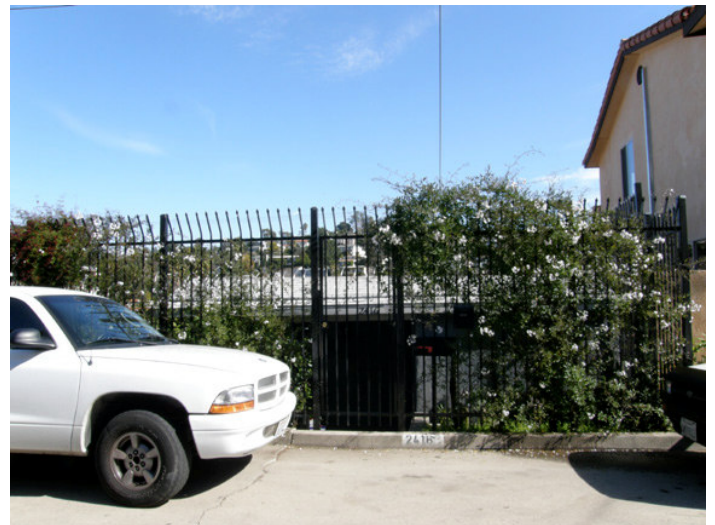
Rear over-in-height fence at 2416 Tracy Terrace
