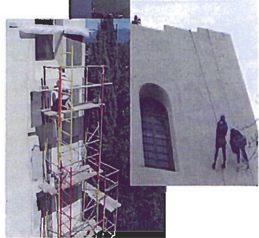
Waterproofing the building
